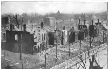
Nashville, Tenn., suffered March 22nd from the most disastrous fire in its history. When the conflagration was checked a strip three blocks wide and nearly a mile long had been burned. This is a typical street after the fire. (By S. A. Weakley)
